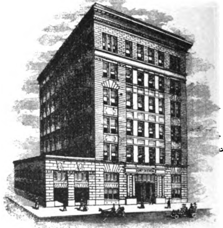
Continental Bank and Trust Company Building, Shreveport, La.
